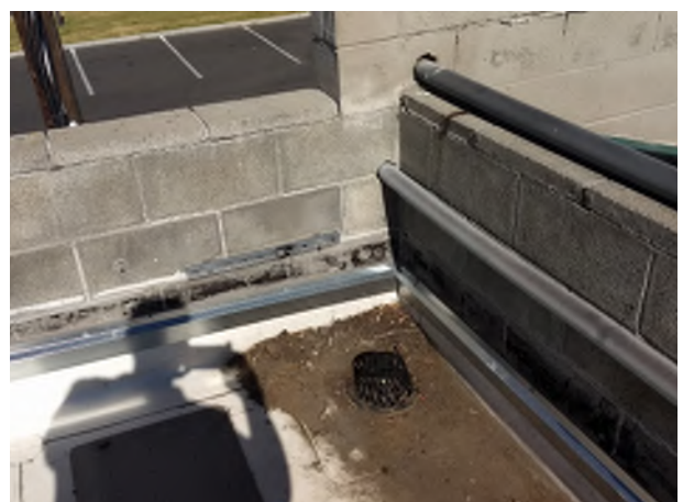
Masonry wall cap, install metal wall cap flashing
