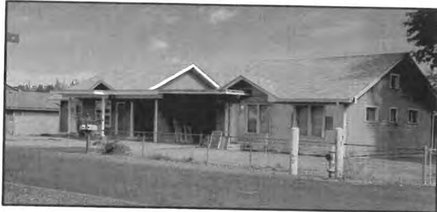
❖ Facing east at Riverview Avenue.
