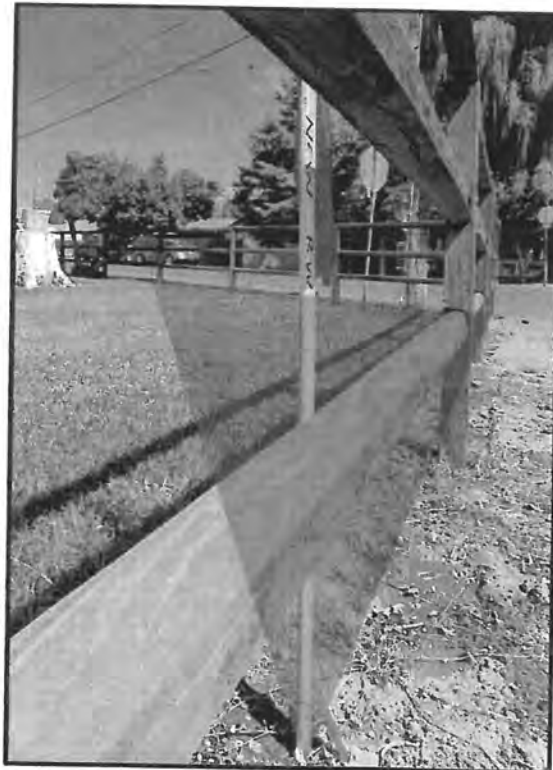
❖ Facing acquisition area at the corner northwest corner of Pleasant Avenue and Third Street.
