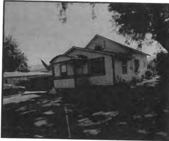
❖ Facing east at Riverview Avenue.
