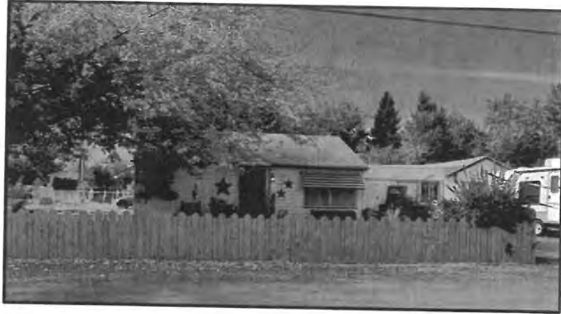
❖ Facing west at Riverview Avenue.
