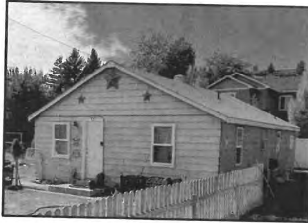
❖ Facing west at Third Street.
