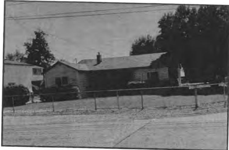
❖ Facing east at Pleasant Avenue.
