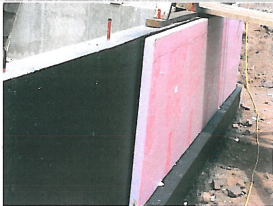
R402.2.8 Basement Walls Exterior insulation R-10 continuous
