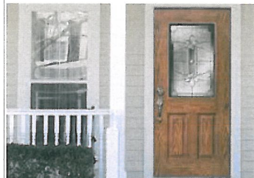
R402.3.4 Opaque Door Exemption One door assembly, up to 24 square feet, is exempt from U-factor requirements.
