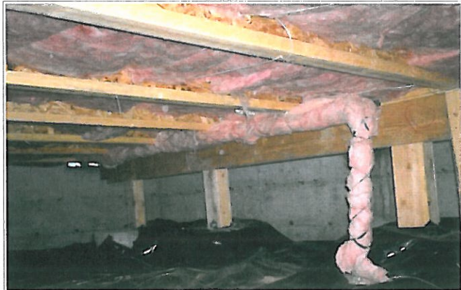
R402.2.7 Floors Floor insulation installed with contact to the underside of the floor decking. Note the inset stapled twine.
