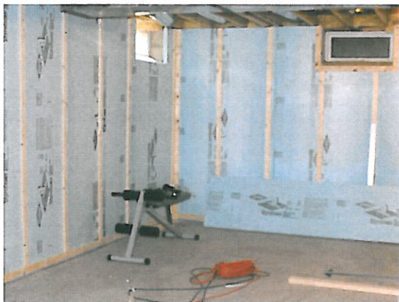
Interior insulation R-15 continuous
