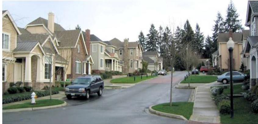
Figure 10.24.120(b)(1) Example of a local access street with integrated parallel parking bulb-outs.
