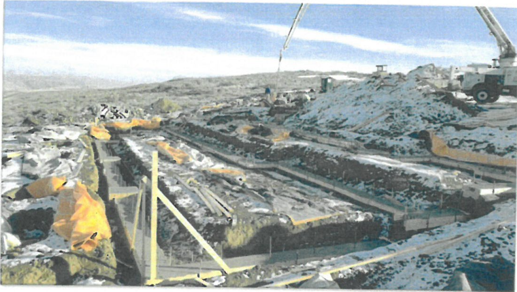
Photo taken by William Longmire of contractor pouring garage footing the same time as house footing on 12/27/2018.
