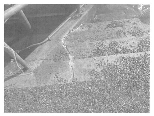
Photo 7: Cracking on access stair. Left side looking upstream.
