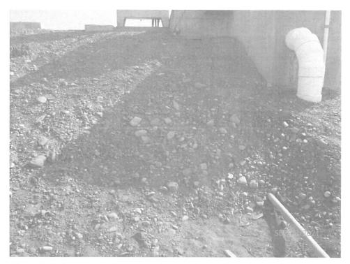
Photo 3: Soil movement on downstream slope adjacent to outlet structure.
