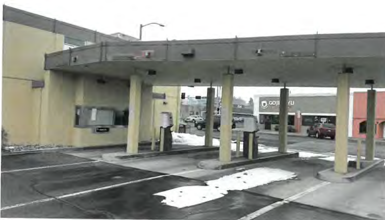
Fascia on drive-thru canopy
