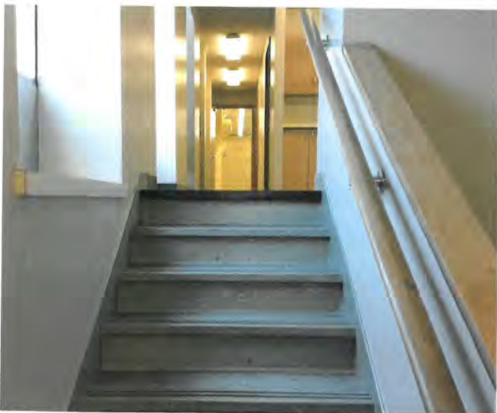
Stairs looking from landing into second floor
