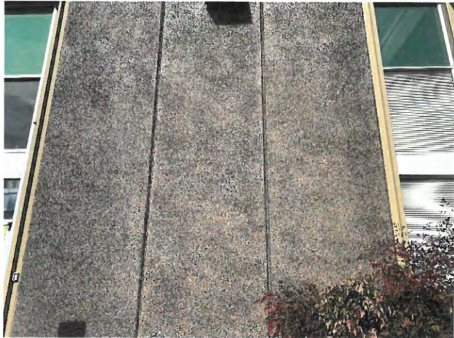
The rock wall with the ACM purple seam sealant
