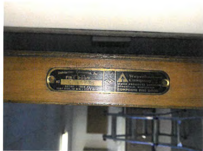
A photograph of the fire door label on the door to the mechanical room.
