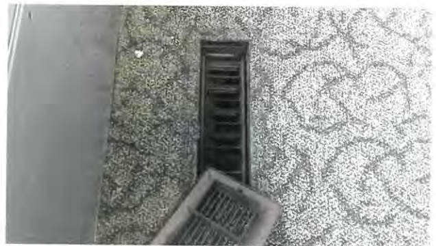
Floor register - First floor
