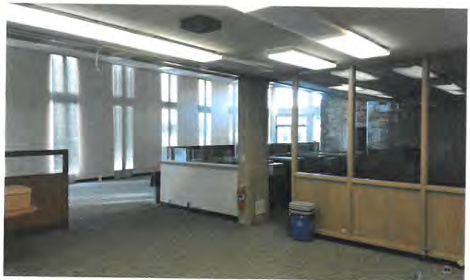
First floor looking northwest
