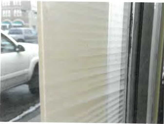
Exterior windows, single pane glazing
