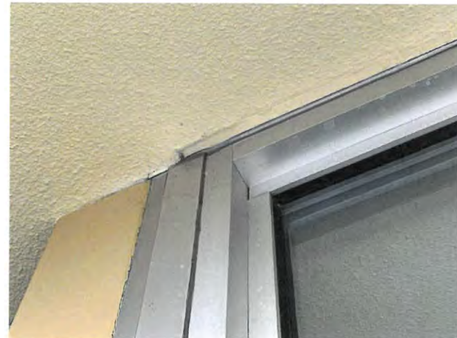
The white putty around textured soffit.
