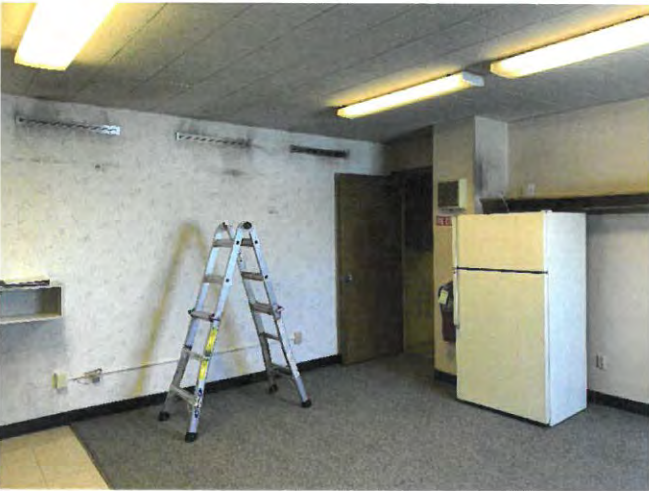
A photograph of the second floor break room. The mechanical room is through the door in the center.
