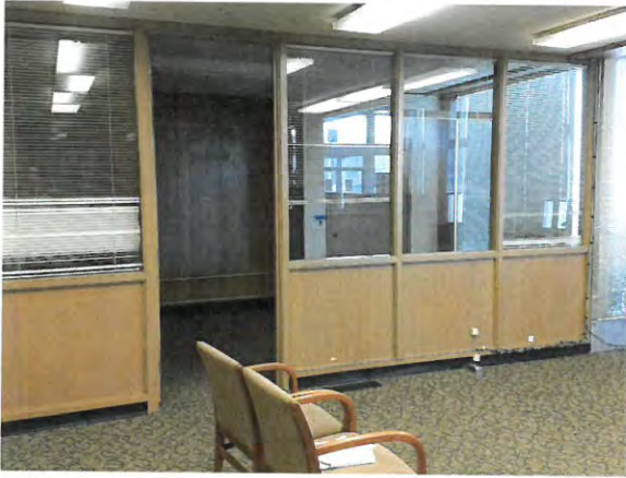
First Floor, office at south end of building
