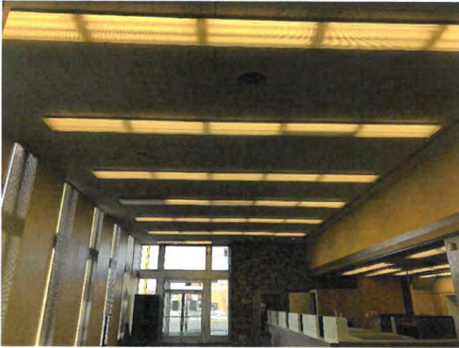
A photograph of the lobby and teller desk. The lighting and electrical systems and 12-inch ceiling tiles with brown glue dots (non-ACM).
