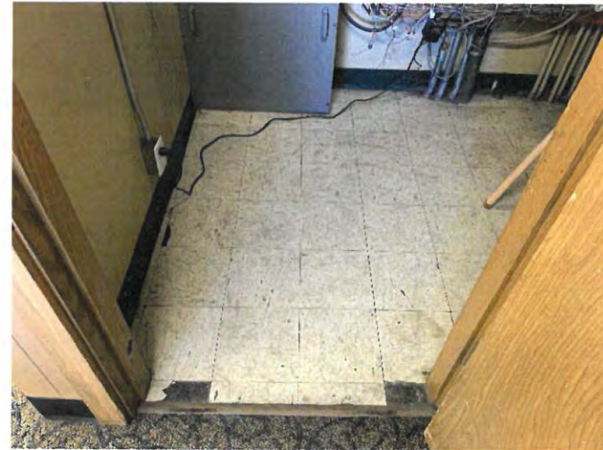
A photograph of the ACM 9-inch off-white vinyl floor tile with speck and ACM black adhesive
