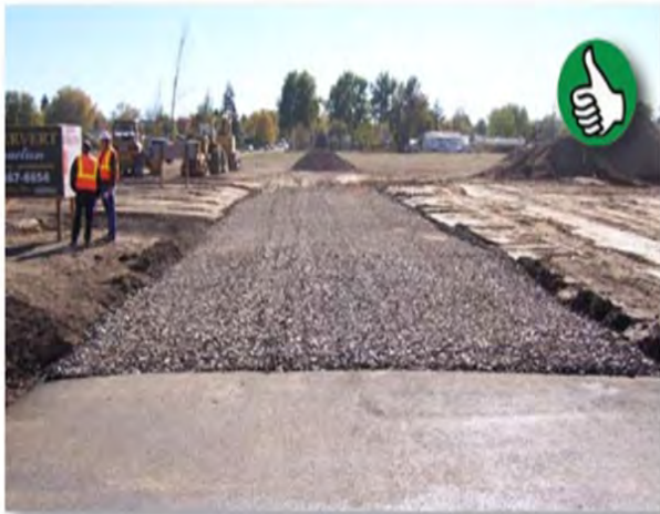
An excellent example of a properly installed construction entrance. (Source: Asotin County)
