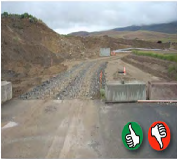
Good installation of a construction entrance, but sediment is still being tracked off-site. Add more rock or make entrance longer. (Source: Douglas County)
